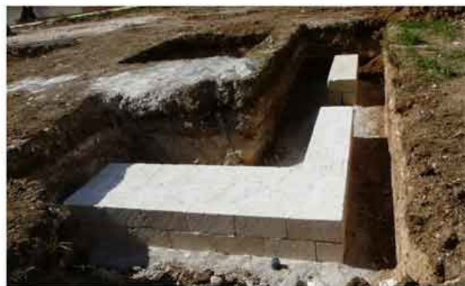
foundation walls in "Leccese" stone
