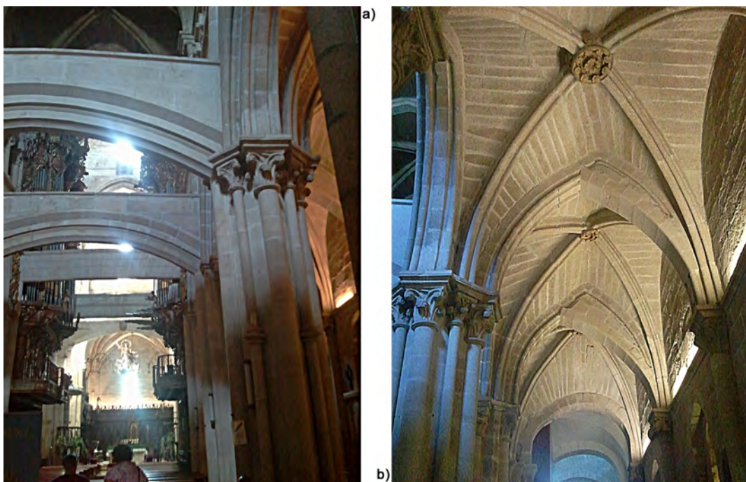
Figure 2-25. Cathedral in Tui (Spain): a) nave and b) lateral aisle
