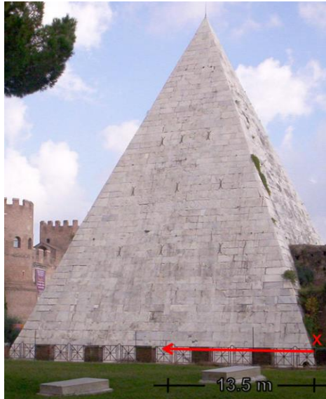
Figure 1.1: Pyramid of Caius Cestius, where the GPR profile path, placed at 1.65 m from the ground level, is superimposed
