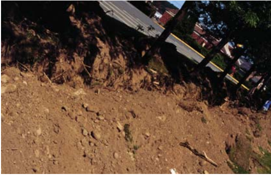
Tree roots are too often disregarded when construction takes place. Great care and planning is required to prevent root damage.
