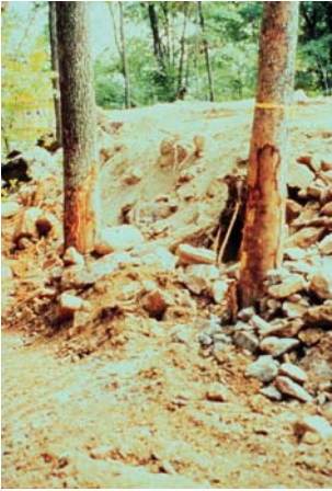
Trees especially trunks and root, are often damaged during construction.
