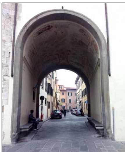
Figure 3 – Detail of “Arco dei Gualandi”.
