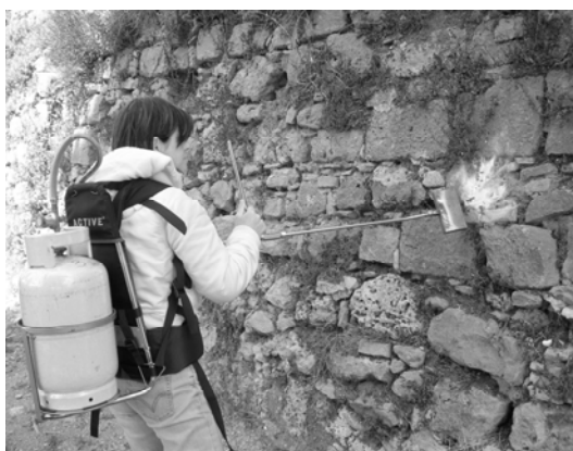
Fig. 3. Flaming on the wall of the Camaldolese Abbey of Volterra by using a backpack flamer.
