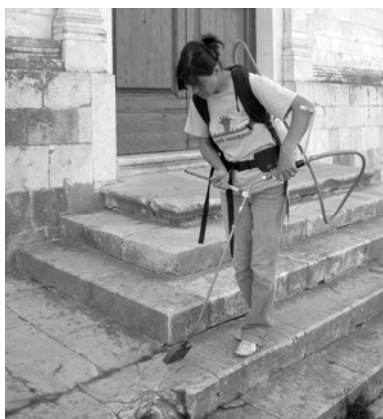
Fig. 2. Flaming on the steps of the SS. Giovanni Battista and Rocco Church of Asciano by using a backpack flamer.
