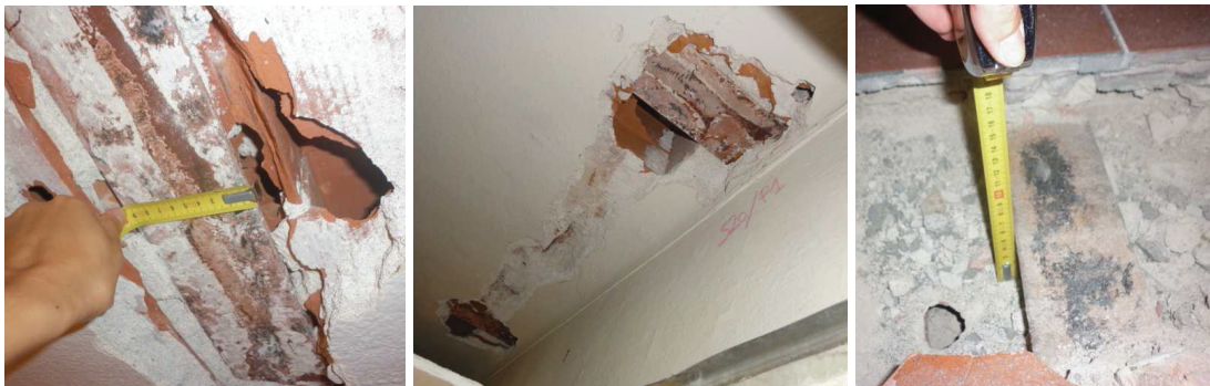
Figure 6: Execution of in situ investigations on horizontal floors with steel elements.
