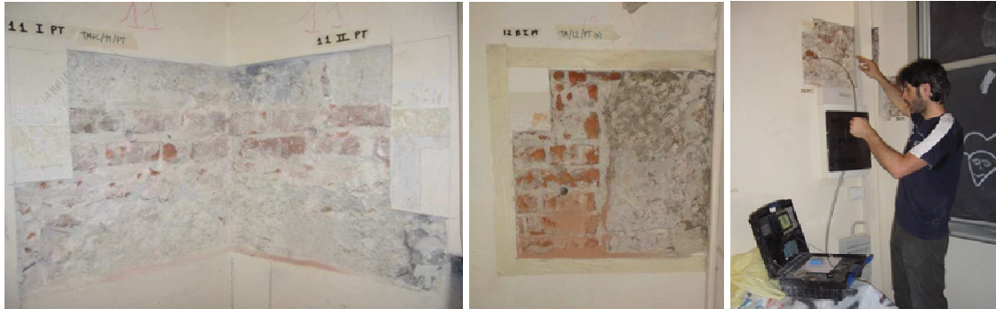
Figure 4: Execution of in situ investigations on masonry walls.
