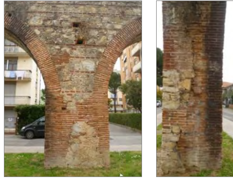
Figure 24 Pillar of arch nr. 130, rebuilt in bricks
