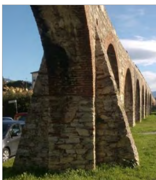
Figure 16 Buttress between arches nr. 89-90
