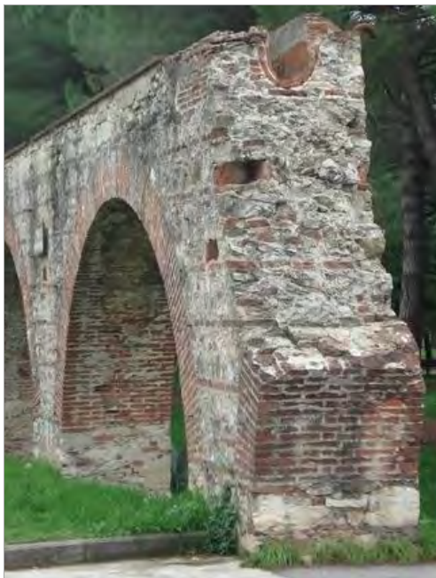
Figure 8 Arch nr. 58, where the core structure and the clay pipeline are visible
