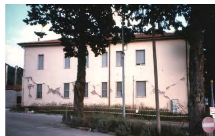
Figure D.3 Diagonal shear cracks in a masonry wall
