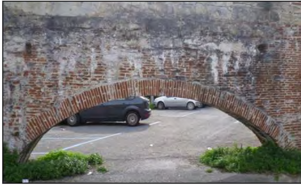
Figure 23 Arch nr. 49, rebuilt in bricks
