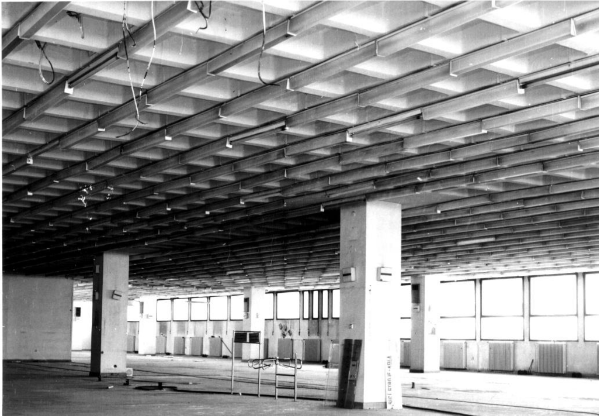
Figure 1 Internal view of the structure
