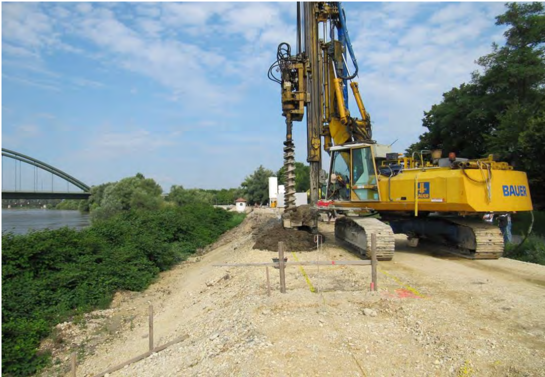
Figure 8 construction of protective levees at the Danube river in Regensburg
