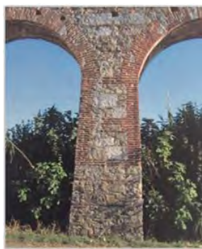
Figure 14 Pillar between arches nr.837 and 838
