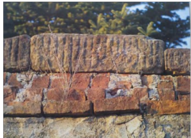
Figure 9 The sheet of stone that covers pipeline
