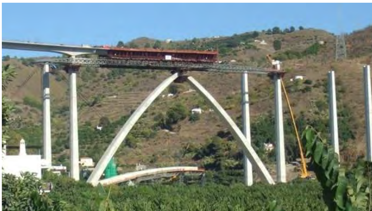
Figure 1 River Verde Viaduct in progress (photograph: F. Nederlof)
