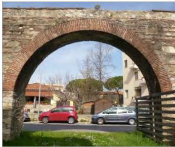
Figure 10 Semi-circular arch (arch nr. 98)
