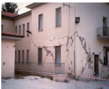
Figure D.3 Diagonal shear cracks in a masonry wall
