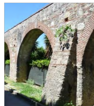
Figure 17 Buttress between arches nr. 199-200
