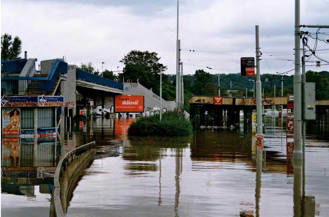
Figure 2 Flooded station of Prague subway system
