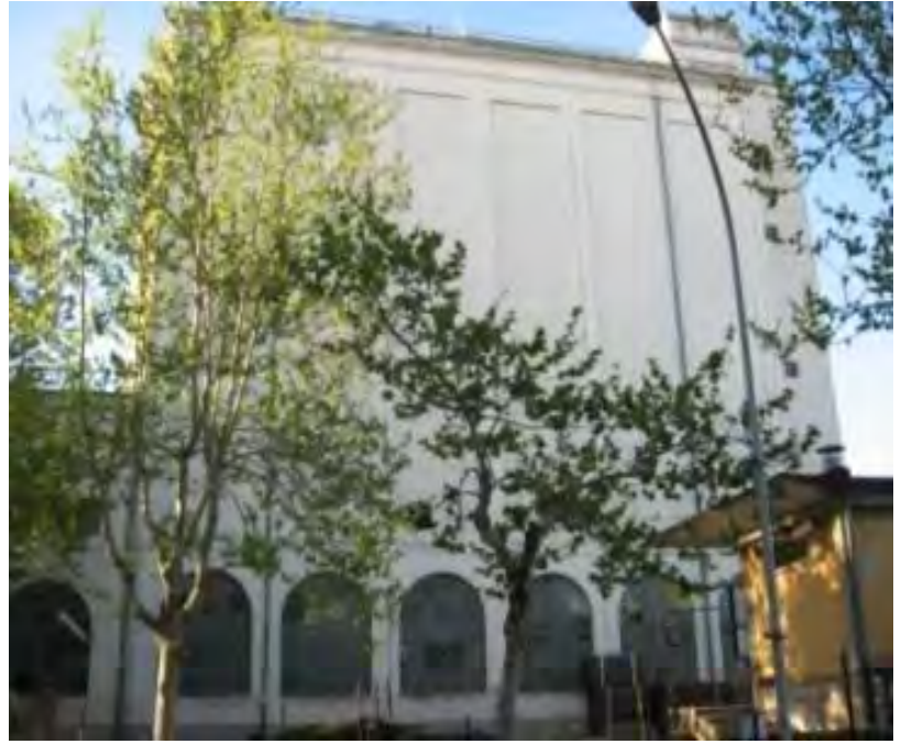
Figure 3 Side view of the silo of the Agricultural Consortium of Grosseto
