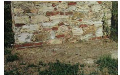
Figure 20 Base under the pillar, between arches n°410-411
