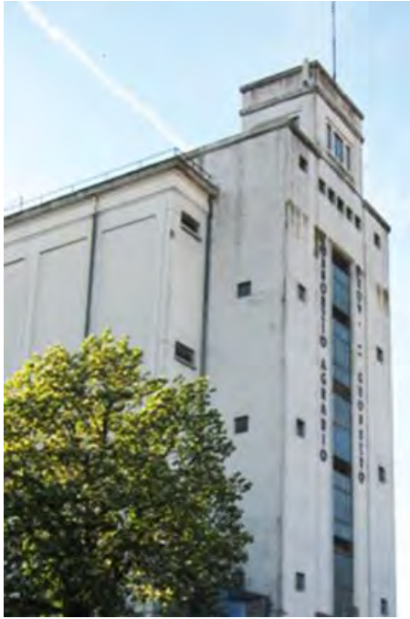
Figure 2 Main façade of the silo
