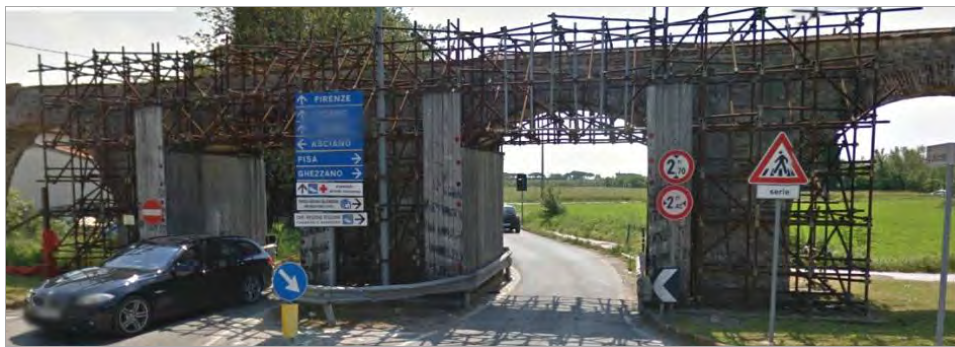
Figure 26 Arches nr. 394 and 395, provisionally supported
