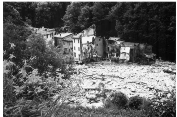
Fig. 4. View of Cardoso village before (a) and after (b) the June 19, 1996 event.
