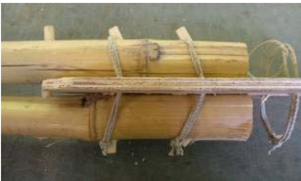
Figure 9. View of a collapsed joint.
