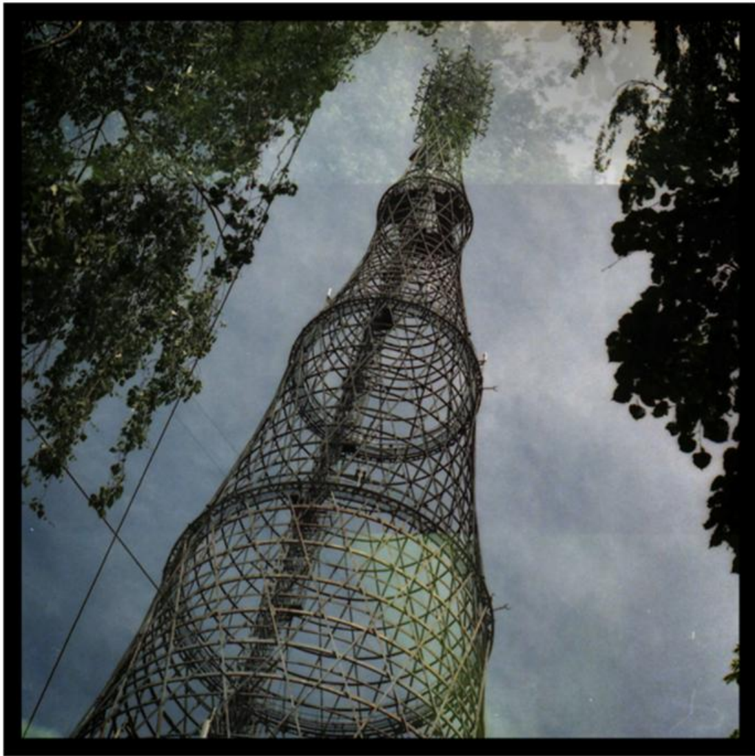
Fig. 3 The Avant-garde radio tower designed by Vladimir Shukhov, 1919-21.
