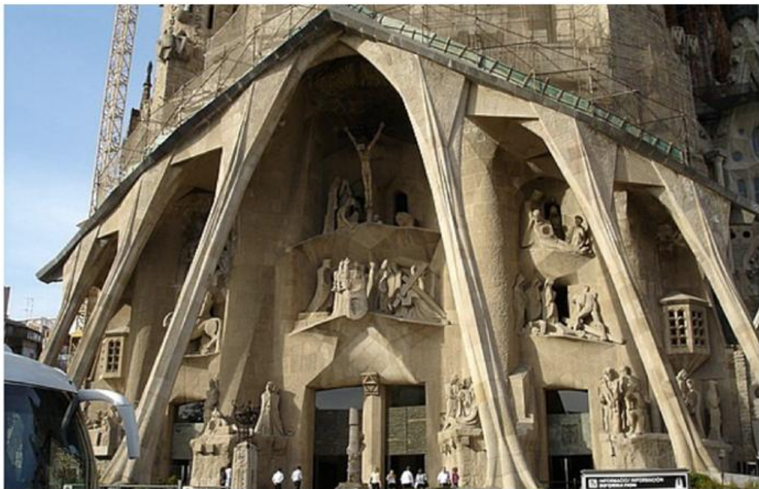
Fig. 2 Inclined hyperbolic columns in the Passion façade of the Sagrada Família.
