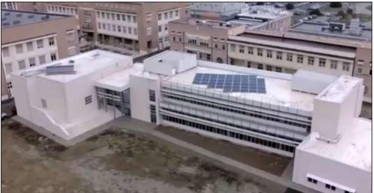
Figure 1. Flat roof with cool white waterproofing membrane (Tecnopolo building of the University of Modena and Reggio Emilia, Modena, Italy).
