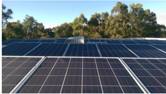
Fig. 3. Partially shaded roof of a building. Different panels are shaded, global production is greatly reduced and investment plan varies.
