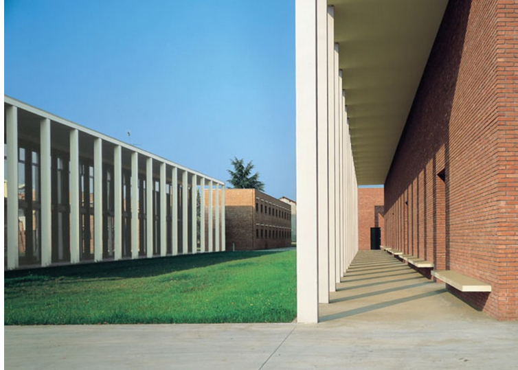
Figure 6. House for elders at Galliate (Novara, Italy), project by Antonio Monestiroli, Alessandro Colbertaldo, Antonio Paolucci, Paolo Rizzato, 1982 - 1989.
