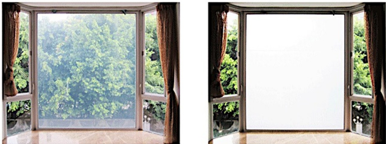
Figure 12. Window with electrochromic glass.
