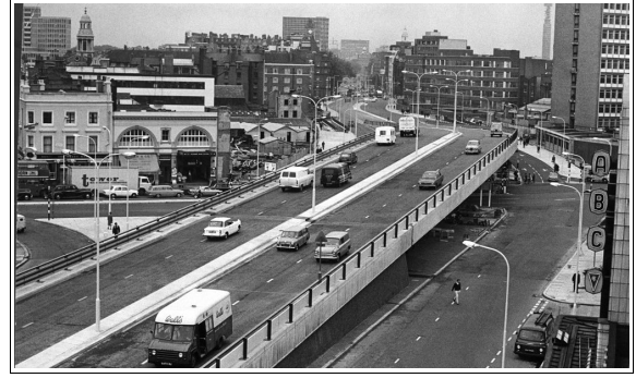
Figure 59. Road elements and relationships with the built environment - London's Edgware Road flyover at its opening in 1967 (source: https://www.theguardian.com/cities/2015/apr/28/end-of-the-car-age-how-cities-outgrew-the-automobile )
