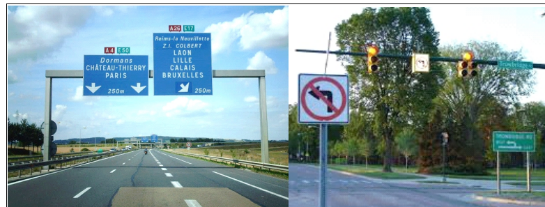
Figure 64. Road equipment /vertical signs, traffic light systems
