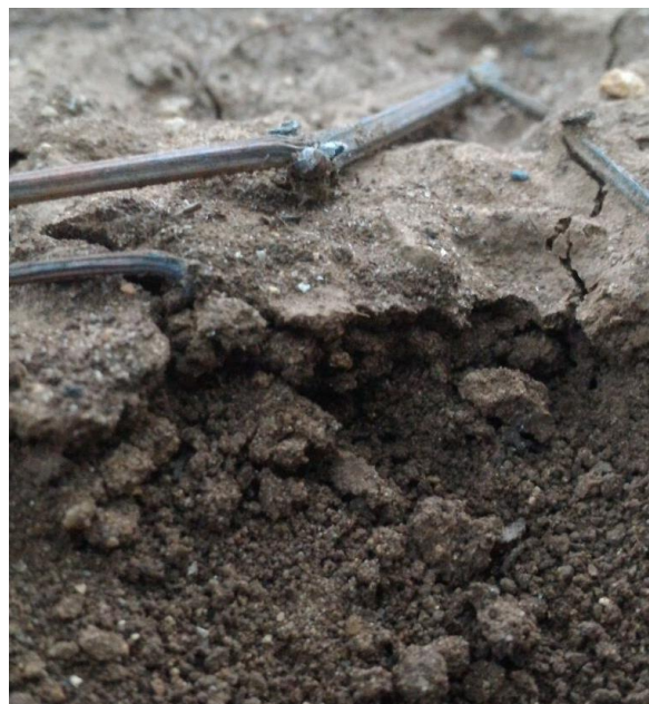
Fig. 2 Surface seal layer developed after the intense storms fallen in September 2015.
