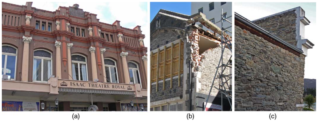
Figure 7. Examples of clay brick and stone URM parapets: (a) clay brick parapet; (b) combination of stone and clay brick parapet; (c) rubble stone parapet.
