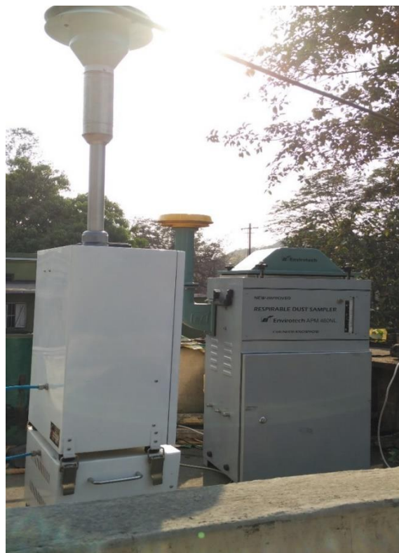
Figure 5.3 Dust samplers installed at Mines Manager's office
