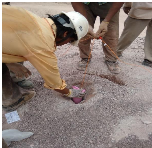
Fig 14: Charging of blast hole with Supergel explosive at Dunguri mine (ACC)
