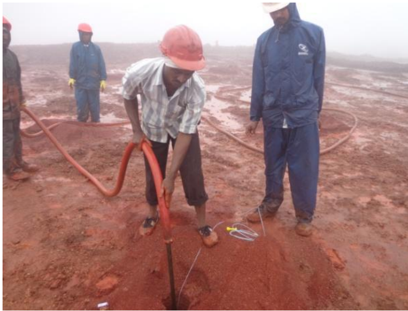
Fig 18: Charging of SME in the blast hole
