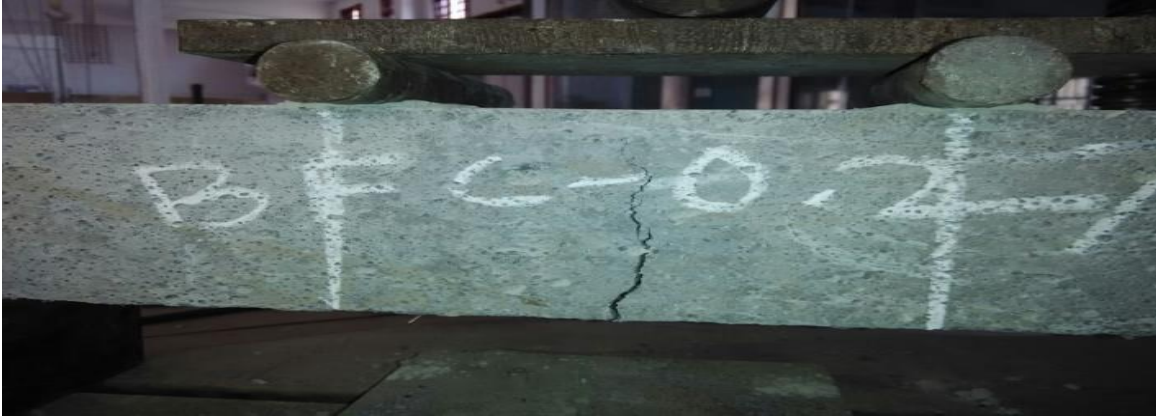
Fig. 4.5.2 Crack Pattern of BFC
