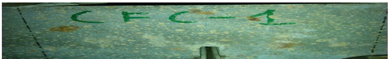
Fig. 4.6.13 Crack Pattern of CFC-1
