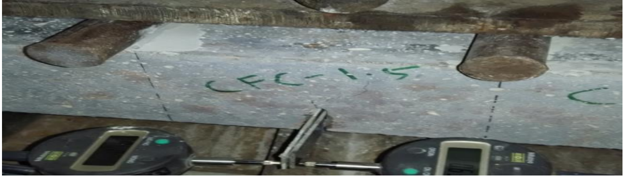
Fig.4.6.14 Crack Pattern of CFC-1.5
