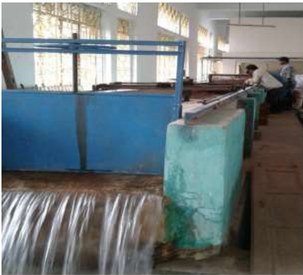
Fig.3.2: Photo of tail gate at downstream.
