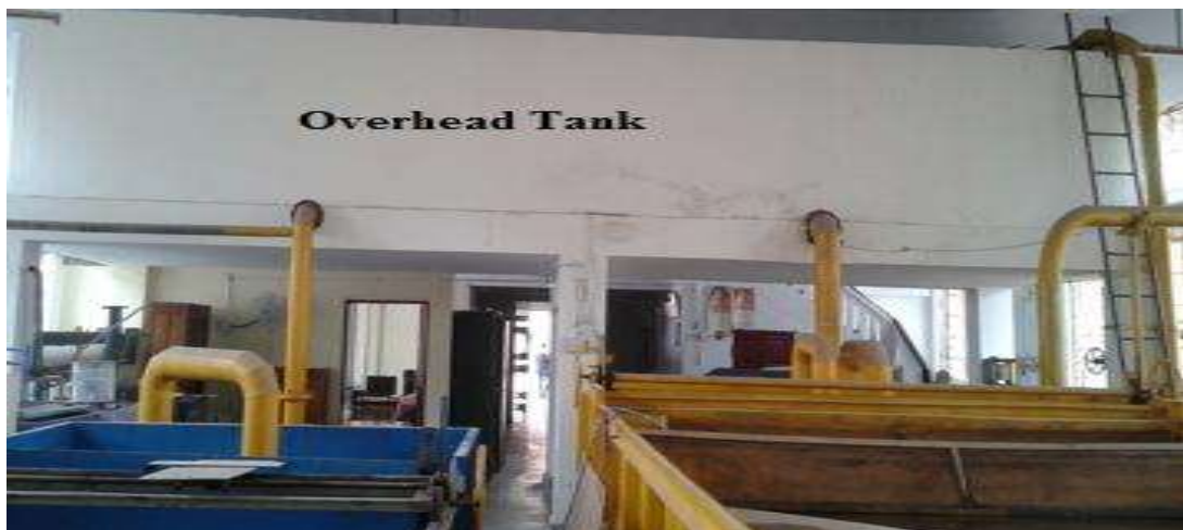
Fig 3.4: Front view of the RCC overhead tank
