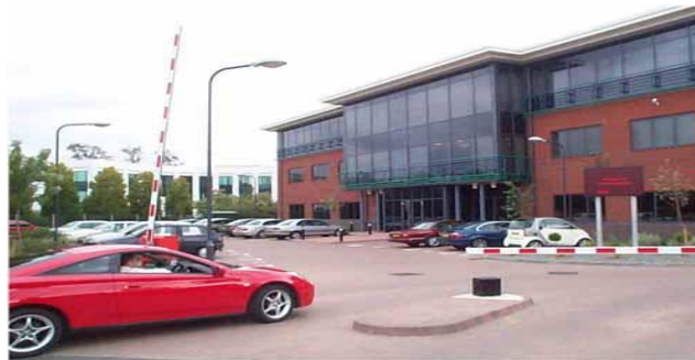
Figure 6.2: ANPR use as access control
