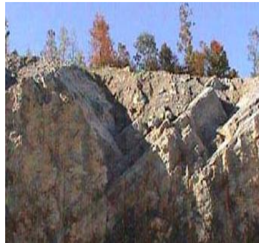
Figure 5: Wedge failure
