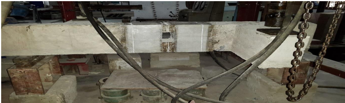
Fig 4.10(b) Crack pattern of BSRO3
