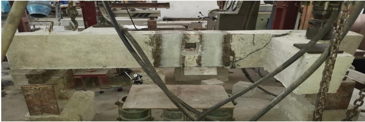
Fig 4.8(b) Crack pattern in BSRO1
