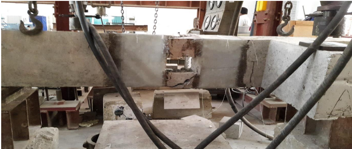
Fig 4.7 Crack pattern in BRO4
