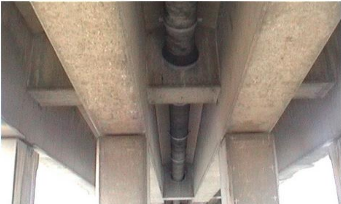
Fig 1.1 Water diversion pipe lines passing through the beams
