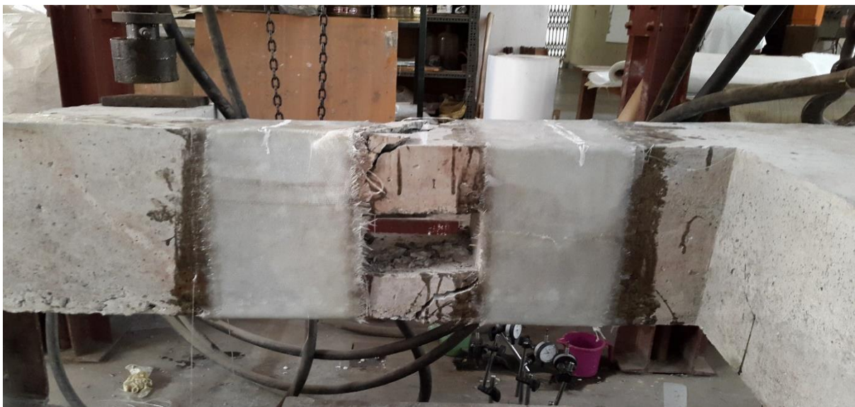
Fig 4.6 Crack pattern in BRO3
