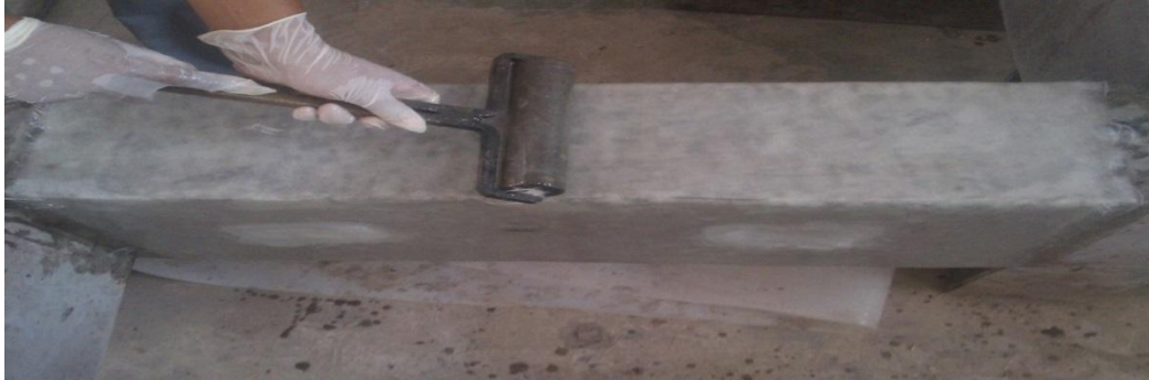
Fig 3.3 Roller Used To Remove Air Bubbles
