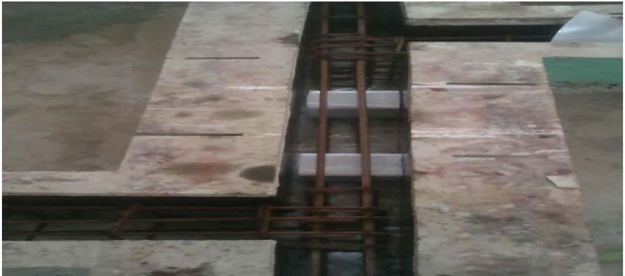
FIG 3.5 Form Work of Beam
