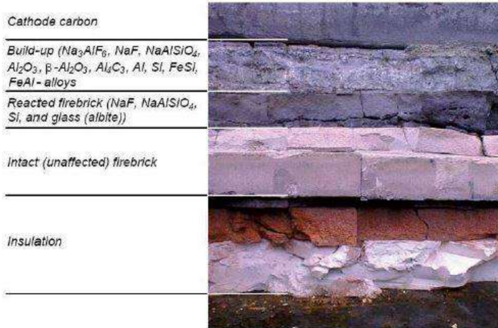
Figure 2.1: Different layers in a cathode bottom lining after 1500 days in operation 44
