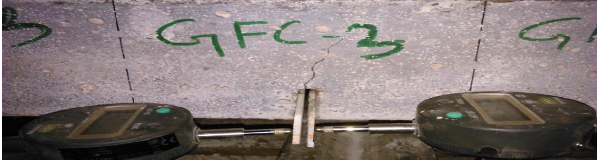
Fig 4.6.5 Crack Pattern of GFC-3
