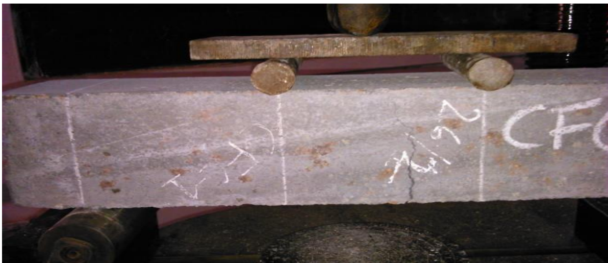
Fig. 4.5.4 Crack Pattern of CFC
