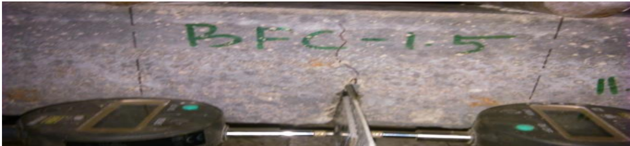
Fig. 4.6.8 Crack Pattern of BFC-1.5
