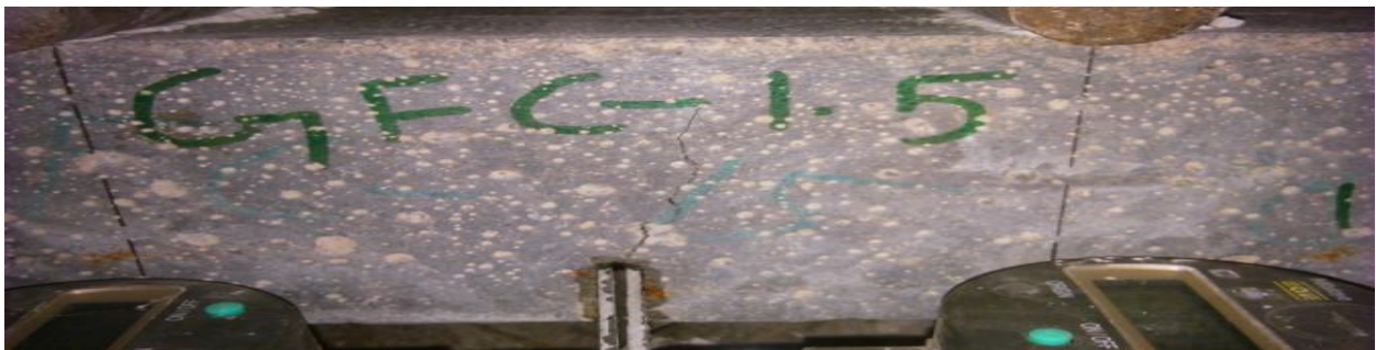
Fig. 4.6.3 Crack Pattern of GFC-1.5
