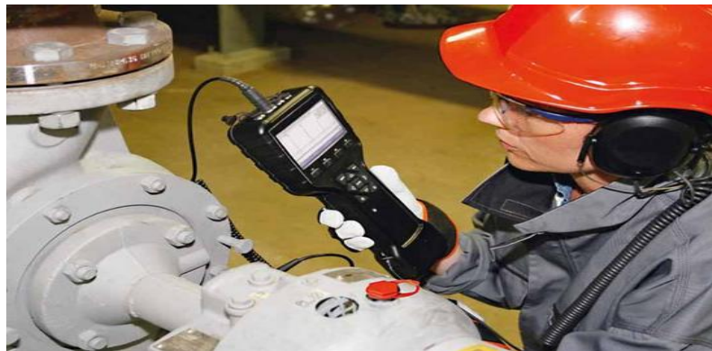
Shock monitoring by shock pulse meter
