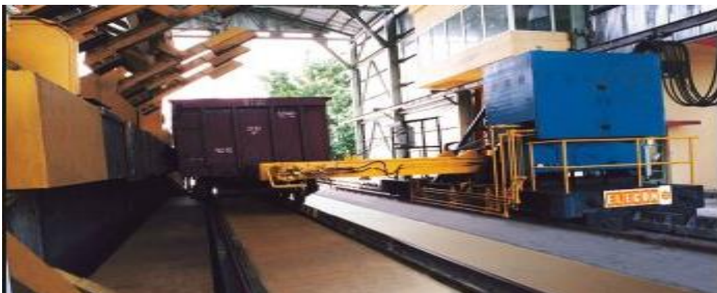
Fig 3.3: A snapshot of Side Arm Charger positioning the wagon in Tippler area.
