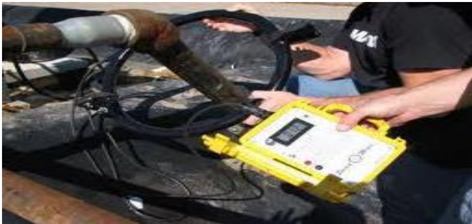
Corrosion monitoring by corrosion meter
