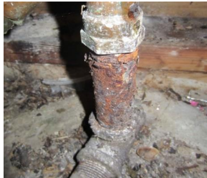
Galvanic Corrosion
