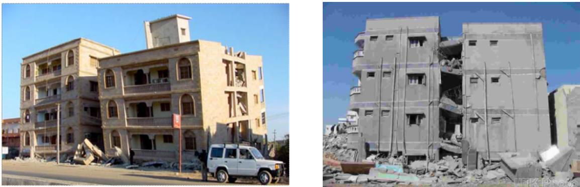
Fig.1.2: Failures of OGS building during 2001 Bhuj Earthquake ([www.nicee.org](http://www.nicee.org))
