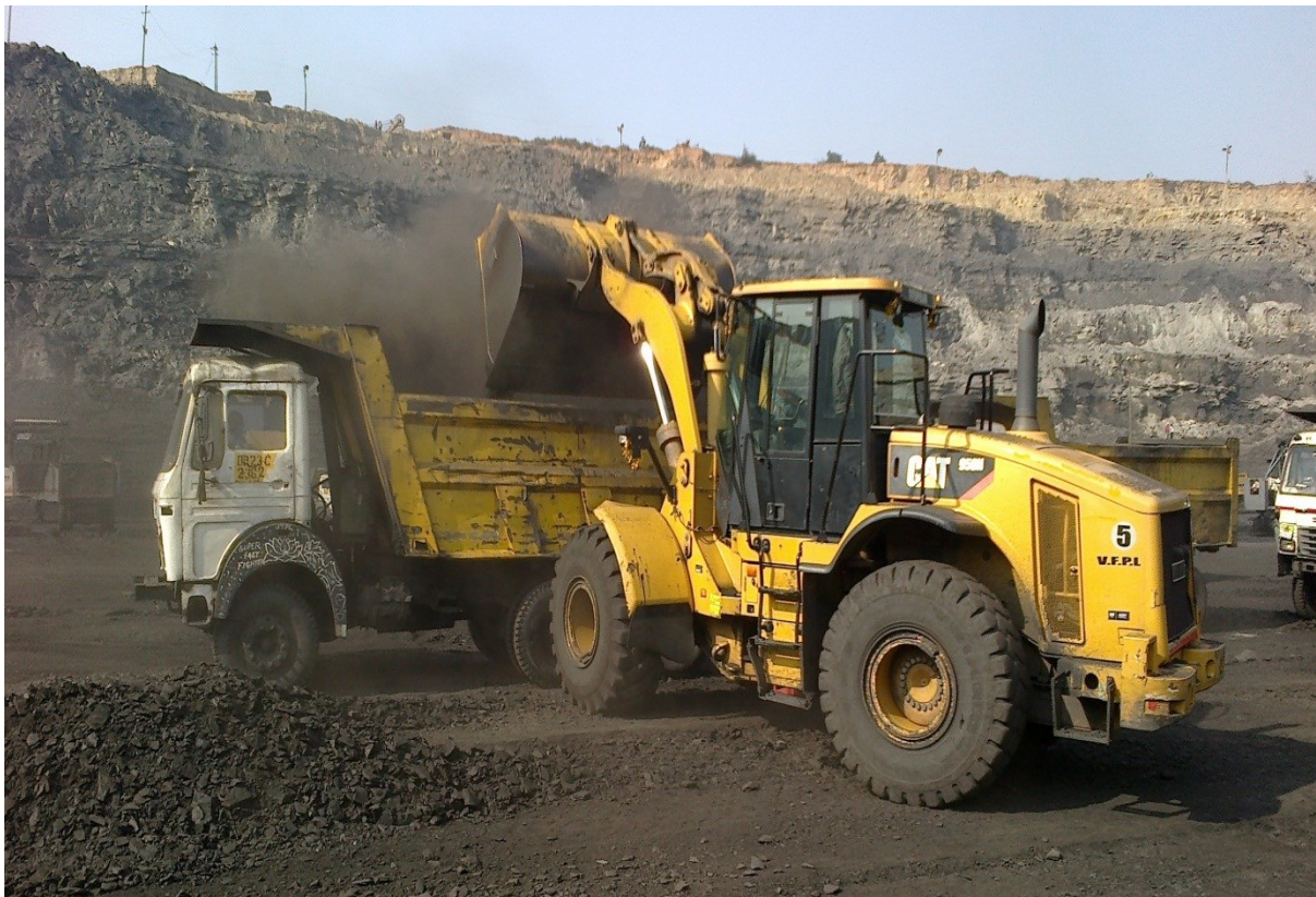
Figure 4.4 Loading point at LOCP for shovel and dumper
