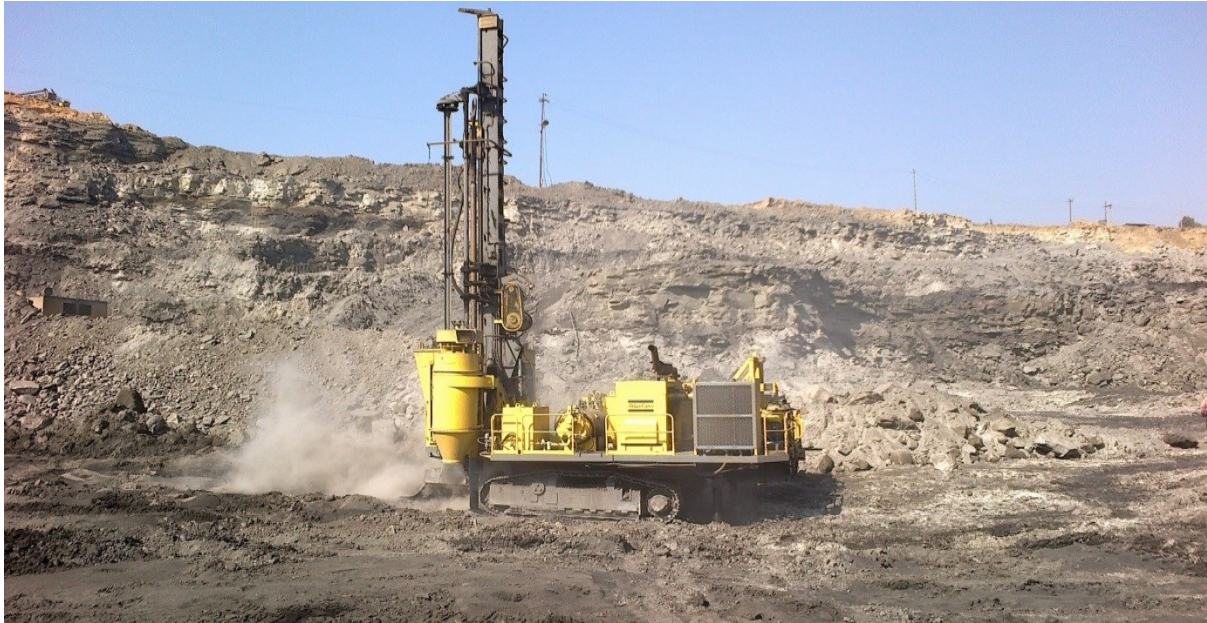
Figure 4.14 Drilling operation at LOCP
