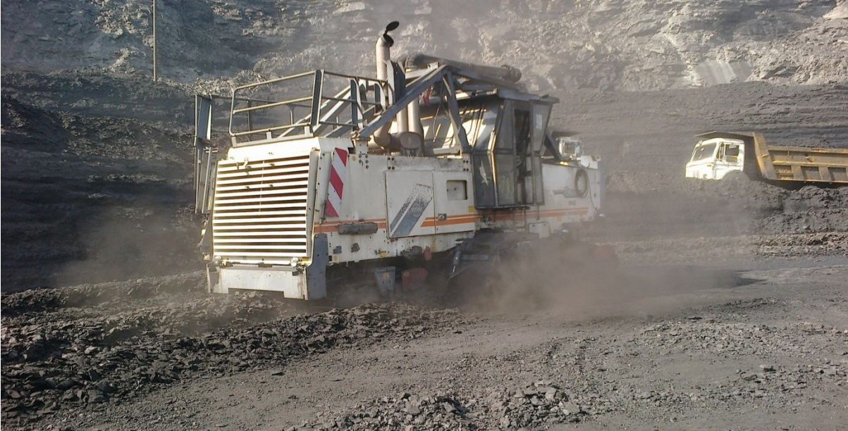
Figure 4.9 Surface miner in operation at LOCP
