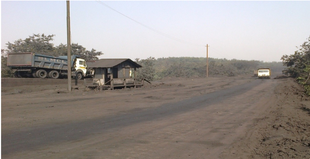
Figure 4.24 Transportation road at LOCP
