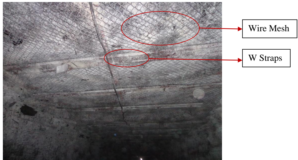
Fig 1.2 Wire mesh supports with w straps in an underground mine[1]
