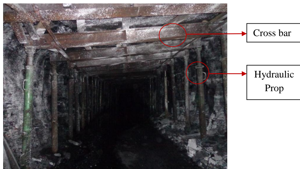
Fig 1.1 Support systems of an underground coal mine[1]
