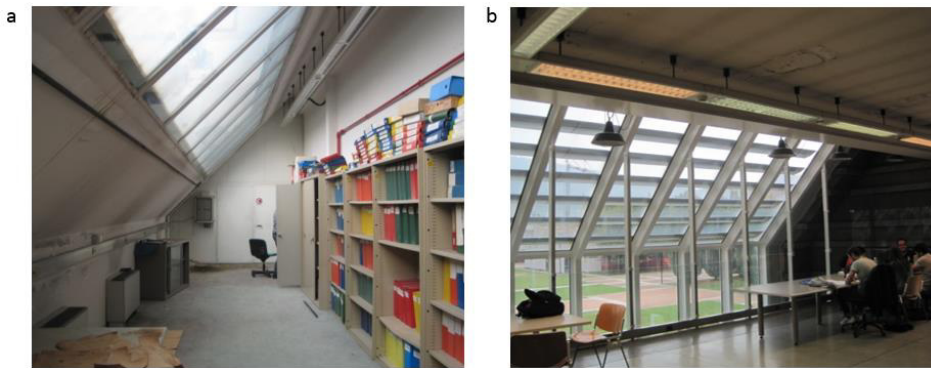
Fig. 2. (a) View of the north-west archive room with the wide window and (b) inside view of the atrium's glazed façade with a vertical portion and a sloped portion.
