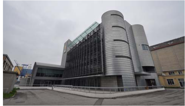
Fig. 5 The examined building.
