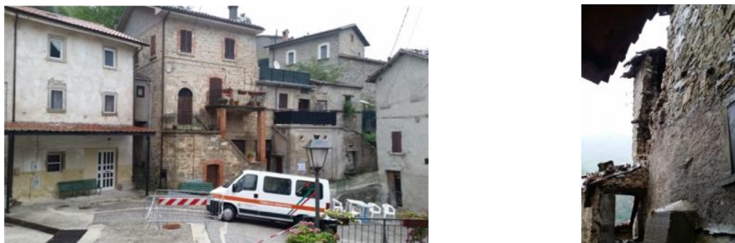
Figure 4: a) Undamaged buildings in the main square of Vezzano village and b) Partial collapse of an abandoned building.
