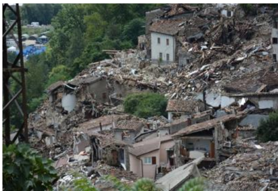
Figure 2: a) Overview of Pescara del Tronto most damaged area and b) Collapse of a typical masonry building.
