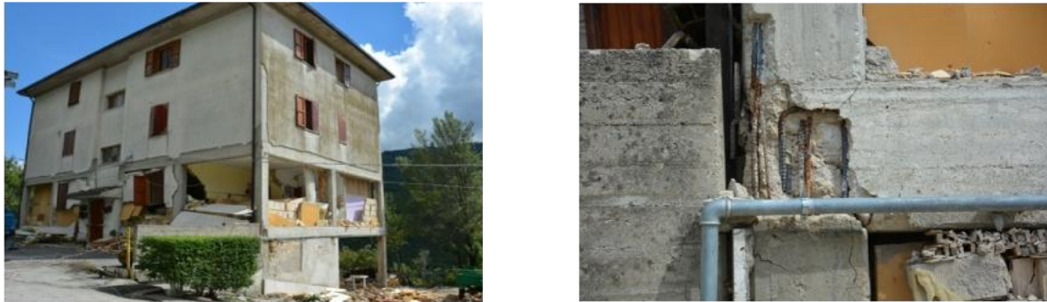
Figure 3: a) Reinforced concrete building in Pescara del Tronto, b) Detail of the damage to a beam-column joint.
