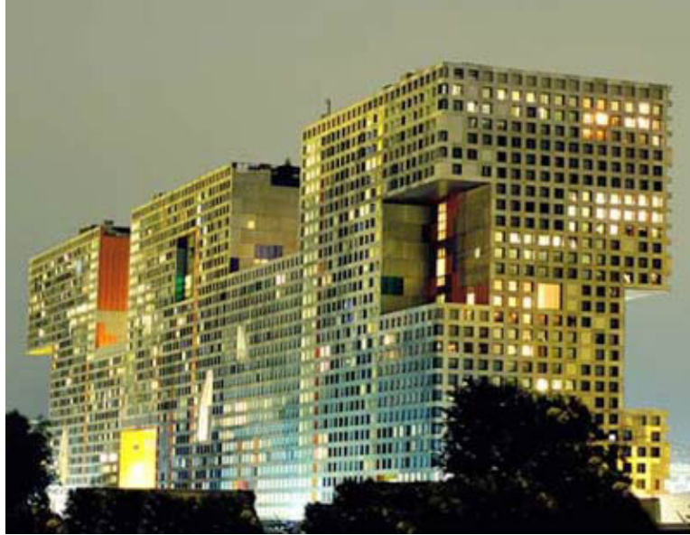
Figure 2: Grid-based design of a façade for Simons Hall in Cambridge, Massachusetts (Architect: Steven Holl, [3]).
