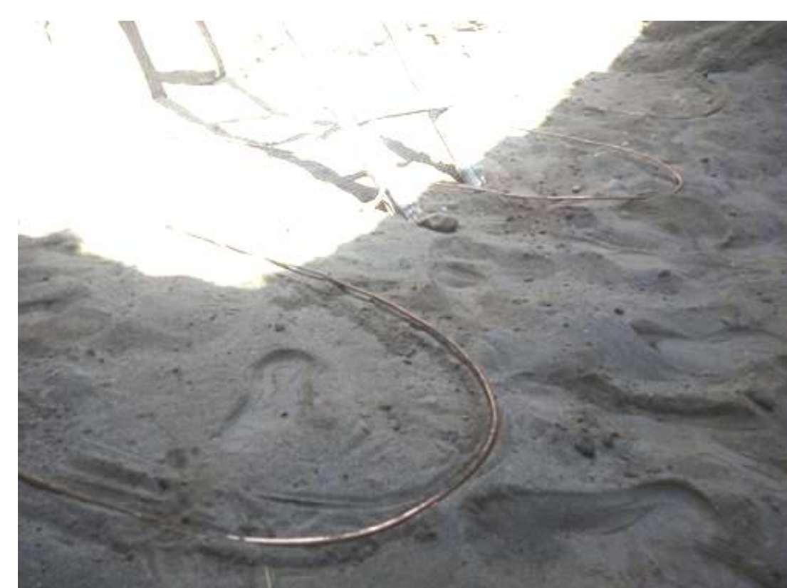
Fig.6 U-loops of copper tubes
