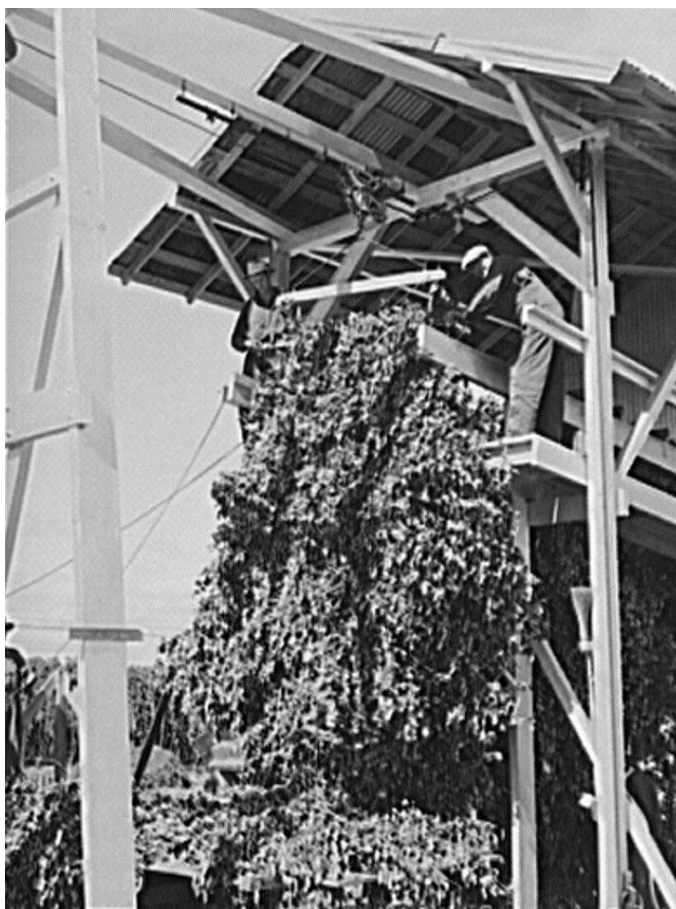
Figure 143. Hop vines going in stationary-type mechanical picker. Putting vines on hooks to begin their journey through the stationary picking machine, where fingers comb hops off the vines. Yakima Chief Hop Ranch. (Russell Lee, 1941), believed to be ~ 1950 or later.
