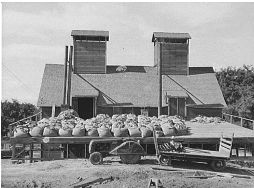
Figure 148. Kiln, sacked green hops in foreground. Yakima County, Washington Double hop kiln still using tall cupolas for natural draft, yet a tractor is employed and the car (left-hand side behind the deck legs) in the picture dates it. (Russell Lee, 1941) LC-USF34-070242. Date may actually be much later.
