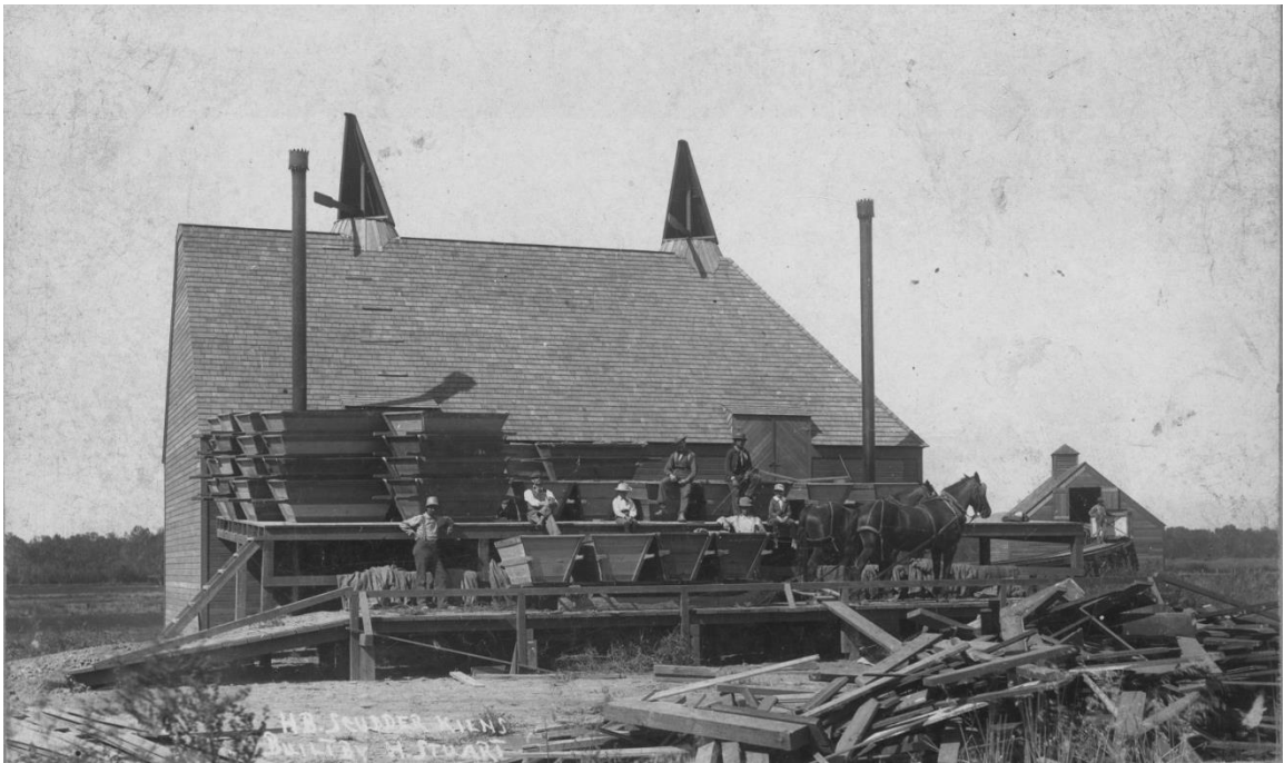
Figure 85. Scudder Hop Kiln, 1905. Location was between West Birchfield Rd. and Gun Club Road, and east of Riverside Road. Notice the building in the background. Looking west, the trees line the banks of the Yakima River. (Margaret Keys Photo Collection)
