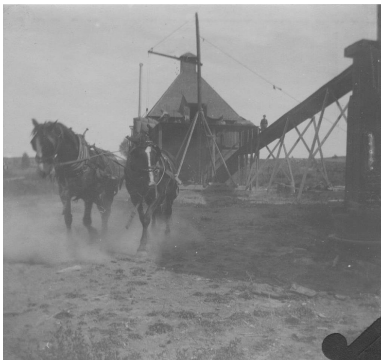
Figure 113. Workers posing on hop kiln. Horse drawn wagon with hop bags in foreground at the Morrier Ranch. The deck of this kiln has no railing. Hops are raised to the deck through horse-power using the hay derrick seen in the photo. You can see two kilns and cupolas in this picture. Date unknown. (Barbara Beane Photo Collection, Yakima Valley Museum, n.d.)
