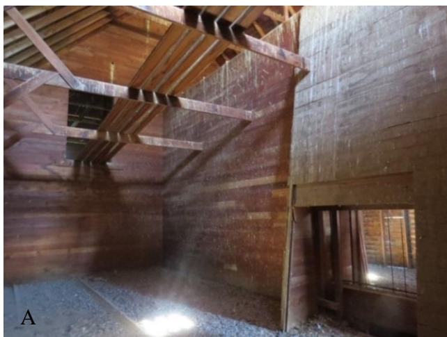
A. The catwalk extends from the drying room to the opposite wall in the cooling room. There is a drying room door on each side of the press, and catwalks on each side. Hops would cool in these rooms and were pushed into the press in the middle when the hops were ready to bale. Gendron Ranch Hop Kiln. (Terri Towner, 2016)
