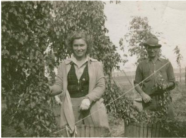
Figure 101. Ferne Heath and her father pick hops in the late 1930s. Slatted wooden and wire hops baskets were used even into the 1950s to pick hops into First was the wooden barrel, then came the woven basket, next the wire frame with a bag attached, and last the wooden slatted basket. (Fern Heath Photo Collection, n.d.)
