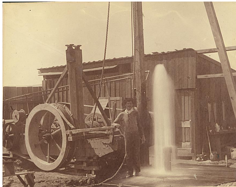
Figure 34. First Artesian Well in Moxee Valley, 1890. Well drilling machine that brought in the first Artesian Well at Mud Springs, 4 miles East of Moxee, in the Yakima Valley. http://www.yakimamemory.org/u?/memory,1617
