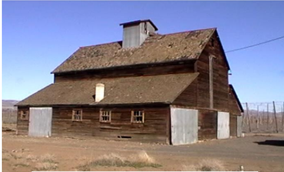
Figure 105. Pete Dufault Kiln on Walters Road, Moxee. It is a single kiln with one cupola and drying room. (Terri Towner, February 2010).
