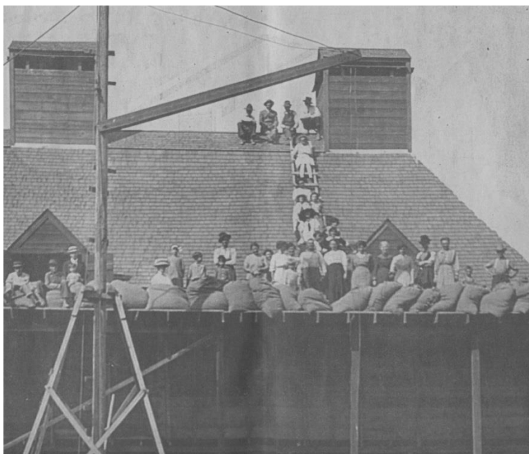
Figure 113. Workers posing on hop kiln. Horse drawn wagon with hop bags in foreground at the Morrier Ranch. The deck of this kiln has no railing. Hops are raised to the deck through horse-power using the hay derrick seen in the photo. You can see two kilns and cupolas in this picture. Date unknown. (Barbara Beane Photo Collection, Yakima Valley Museum, n.d.)
