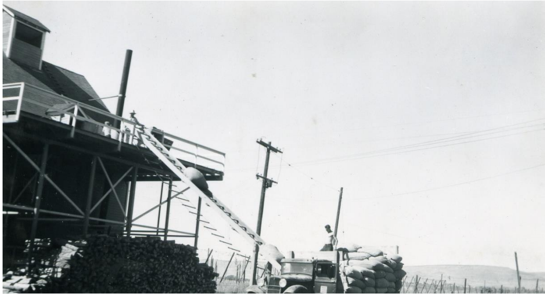
Figure 5. O. J. Gendron Ranch Hop Kiln after 1934. Putting bags of hops up the elevator to the deck and entrance to the drying floor of the Kiln. (Gendron Photo Collection, n.d.).
