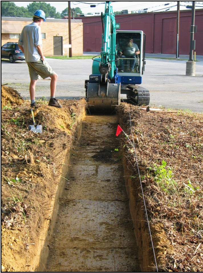
Figure 4. Excavation and Monitoring Trench 5. Facing north.
