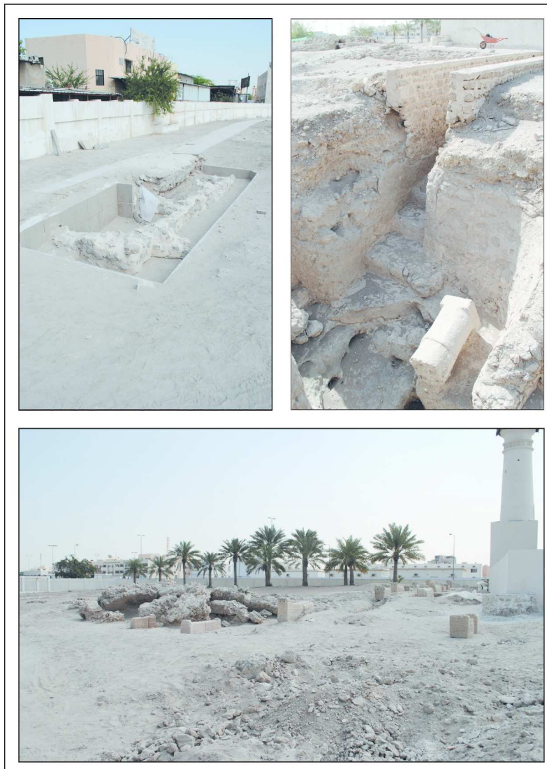
Figure 18. Al-Khamis Mosque site. Left. The well (Area B) with fallen column base in-situ. Right. The multi-roomed building (Area D), after conservation. Bottom. The collapsed shrine (Area A), after conservation (photos. T. Insoll) 193x268mm (300 x 300 DPI)
