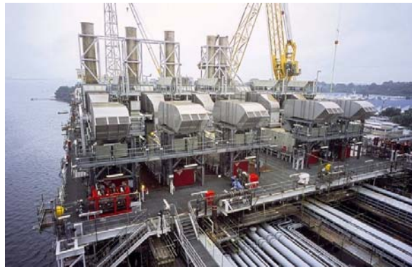
Figure 14: Gas Turbine Installation on an FPSO
