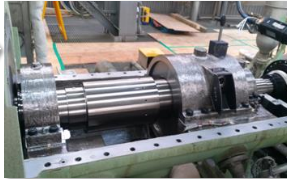
Replacement of DE Journal Bearing
