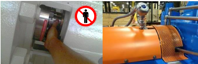
Figure 1: Unguarded shaft area vs. guarded
