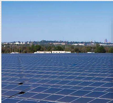
Blue Wing Solar PV Array ,San Antonio
