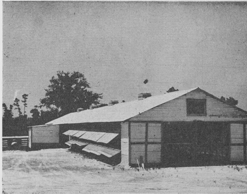
Fig. 3 A recommended type of house. The feed room is situated in the center of this house. Locate yours for convenience in your planned layout and system of feeding.
