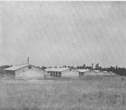
Fig. 1 Locate your houses for convenience, air drainage and sanitation. These houses are arranged so that they do not block off breezes and so that possibility of contamination from one to another is reduced.
