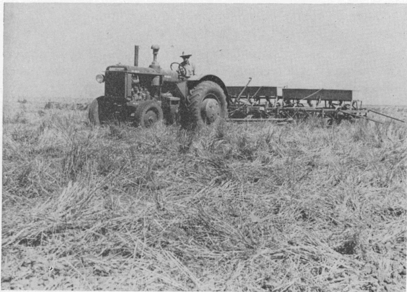
Figure 4. A deep furrow type drill operating in heavy stubble.
