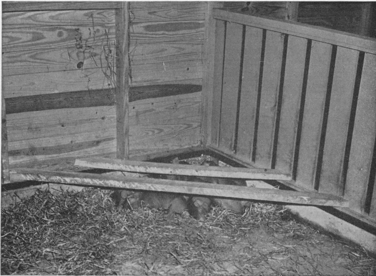
Corner Guard Rails
