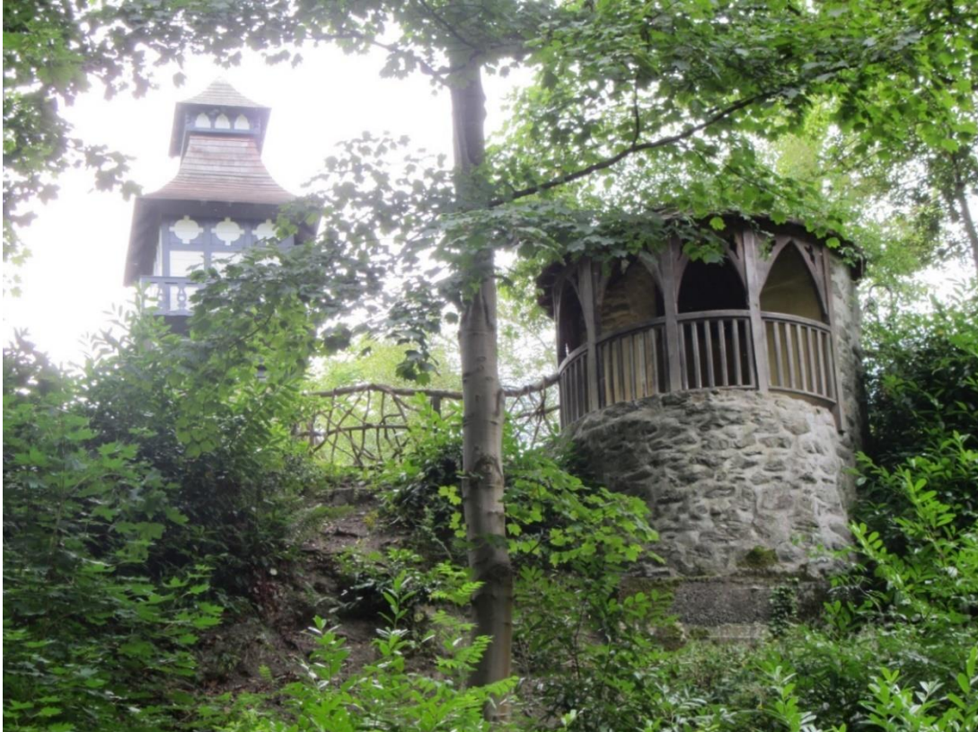
Fig. 68. Not all current structures at Plas Newydd today are original to the landscaping projects that Sarah Ponsonby and Eleanor Butler implemented. This turreted overlook above the gardens below has been built from the foundational hardscape from Eleanor Butler’s bower, but the upper portion is a recent reconstruction. Reprinted from my personal photograph (“Deborah Pfuntner” 2012).
