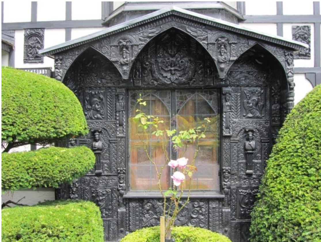
Fig. 66. Plas Newydd library bay window in which found, given, or commissioned carvings from Gothic interiors form the facade design. Reprinted from my personal photograph (“Deborah Pfuntner” 2012).
