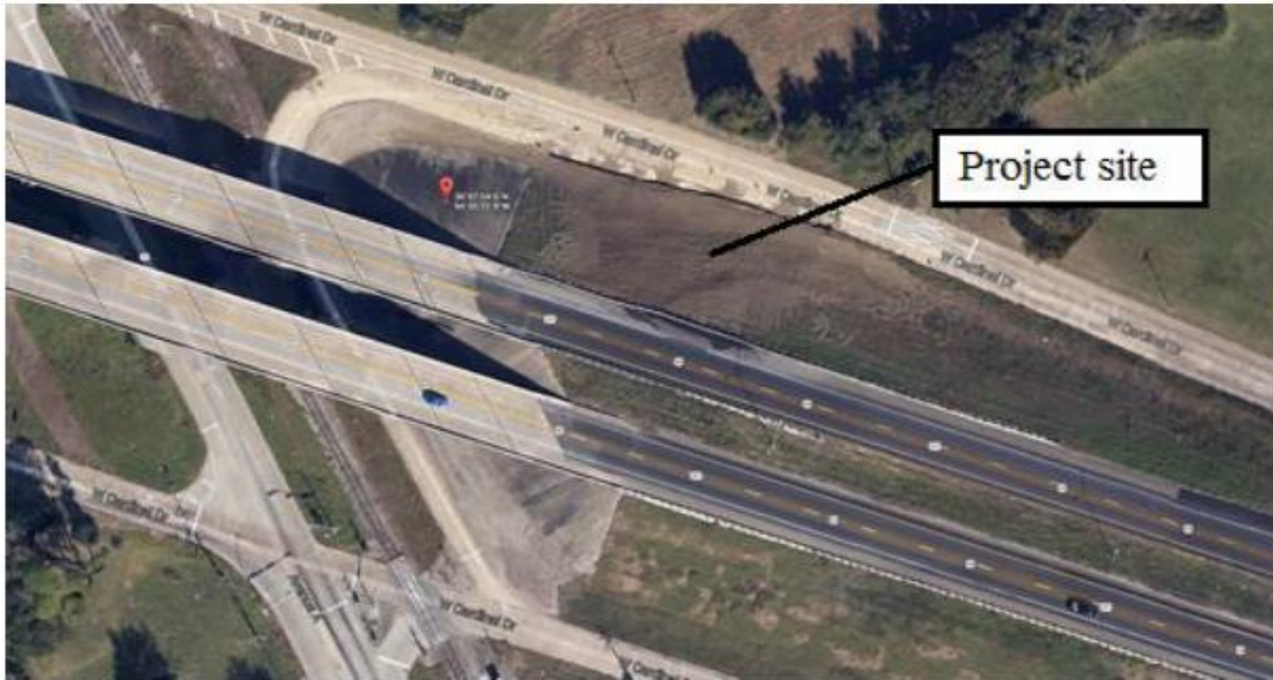
Figure 18 Aerial view of the Beaumont project site after Kharanaghi (2015).
