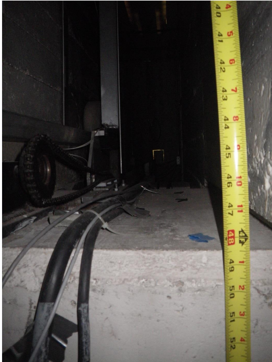
Figure 38. Measurement of the height of the perpendicular portion of the radiography cave.
