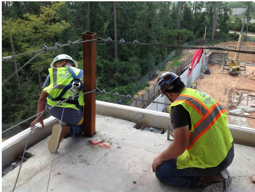
Figure 28. Sill rail installation process. Image: Andres Martinez.
