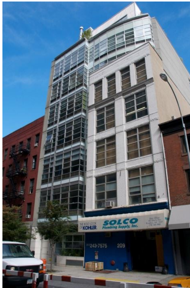
Figure 1. The stick curtain wall system. 211 W. 18 th Street. New York, NY. Image: Andres Martinez.
