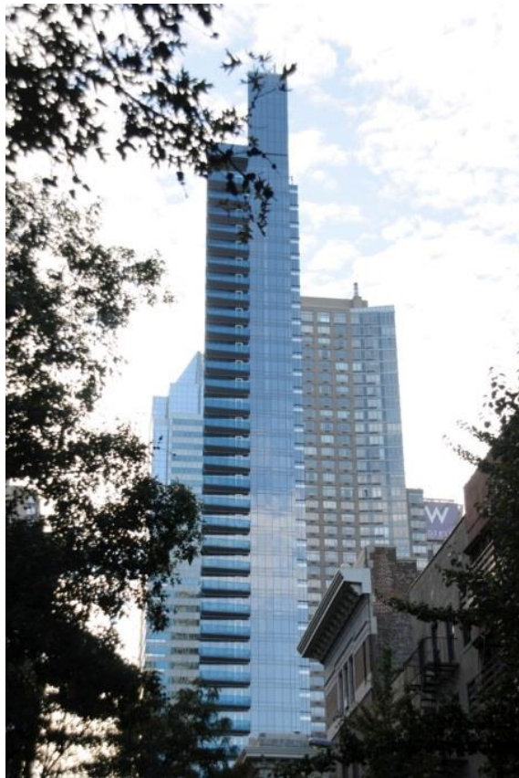
Figure 4. Unitized curtain wall system. 8 th Avenue, New York, NY. Image: Andres Martinez.
