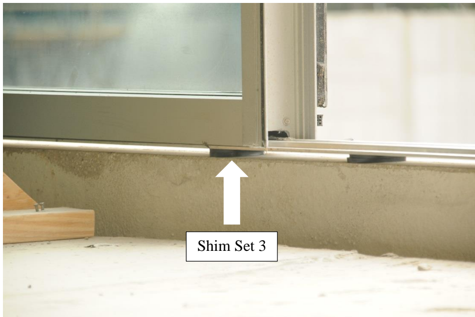
Figure 34. Detail of sill rail leveled with shim set 3. Image: Andres Martinez.
